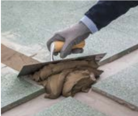
Filling a cable run with Planipatch Xtra
